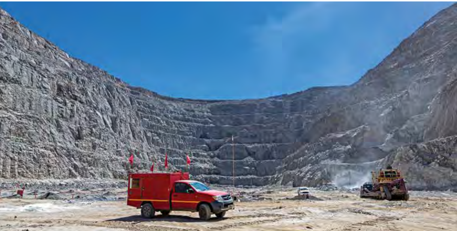
Blasting preparations underway in the open pit.
